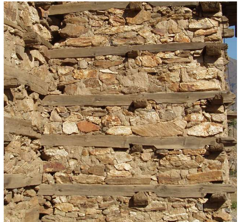
Traditional Bhatar construction Besham Fort (c. 1750) NWFP - Pakistan
